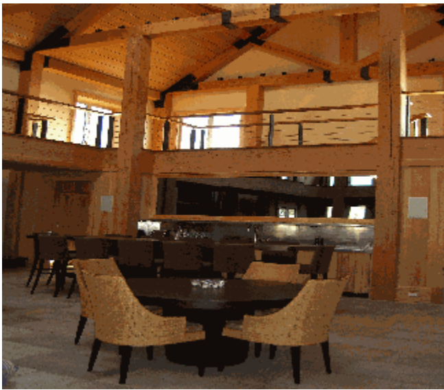
Figure 1. Example Room Two Installation. In this application a high tech 1/32" fiber free absorber was attached to the beams. Planks of wood were then placed on the ceiling joists with a 3/8" space between each plank. The reverberation time of the room without this treatment was such that speech from the media system would have been difficult to understand. Instead the wood spacing described reduced the reverberation time so that the audio system had pure tones and speech was audible
